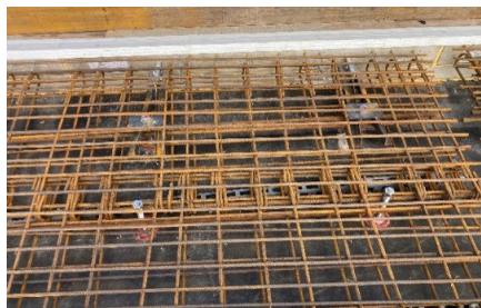
b) Anchors in rebar before pouring concrete
