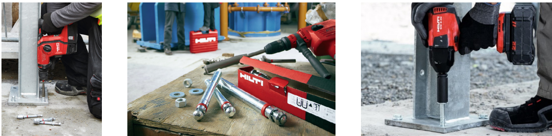
Fig. 8.9: Installation of mechanical anchors using setting tools and impact wrenches
