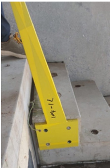
a) Baseplate application during construction
