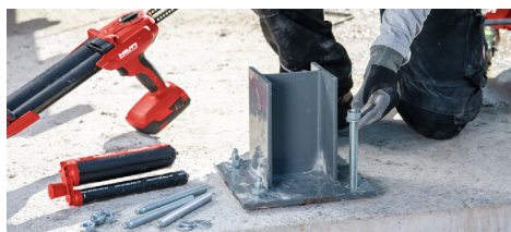
a) Anchors installed in vertically downward direction
