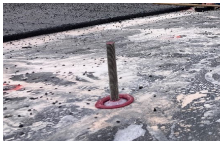
c) Rod with HIW-SD sealing cap for waterproofing
