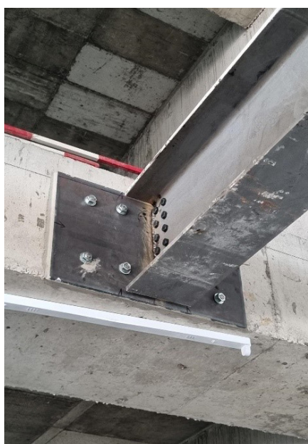
c) Detail of steel to concrete connection
