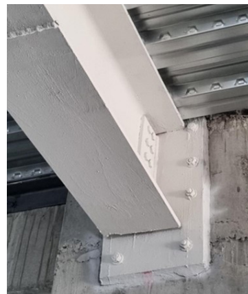
Fig. 6.11: Baseplate connection using group of anchors (4x2)
