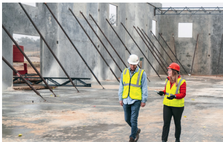
a) Temporary wall support
