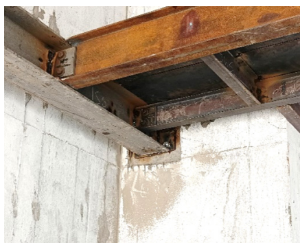
b) Post-anchoring application for baseplate connection
