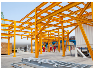
a) Primary steel column
