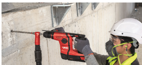
b) Drilling being done for horizontal application
