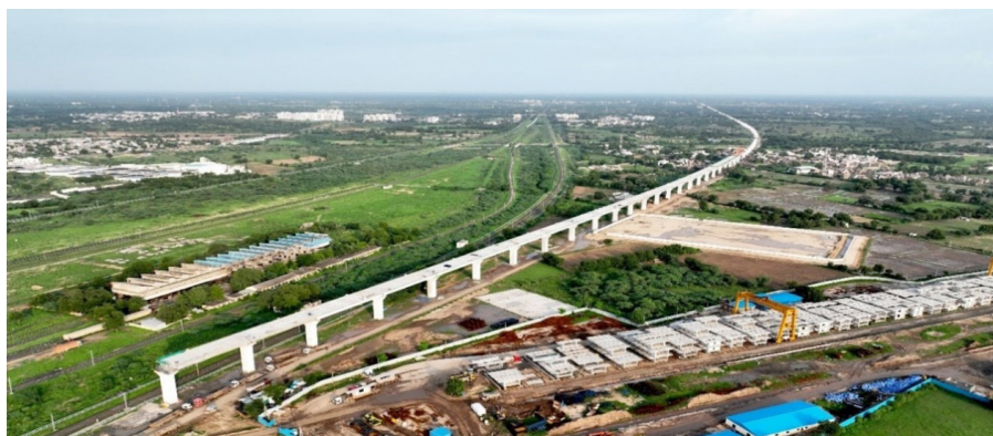
a) MAHSR viaduct portion
