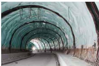
a) Road tunnels are highly corrosive environments
