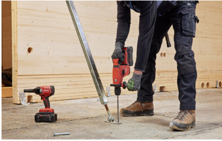
a) Drilling holes with a Rotary hammer
