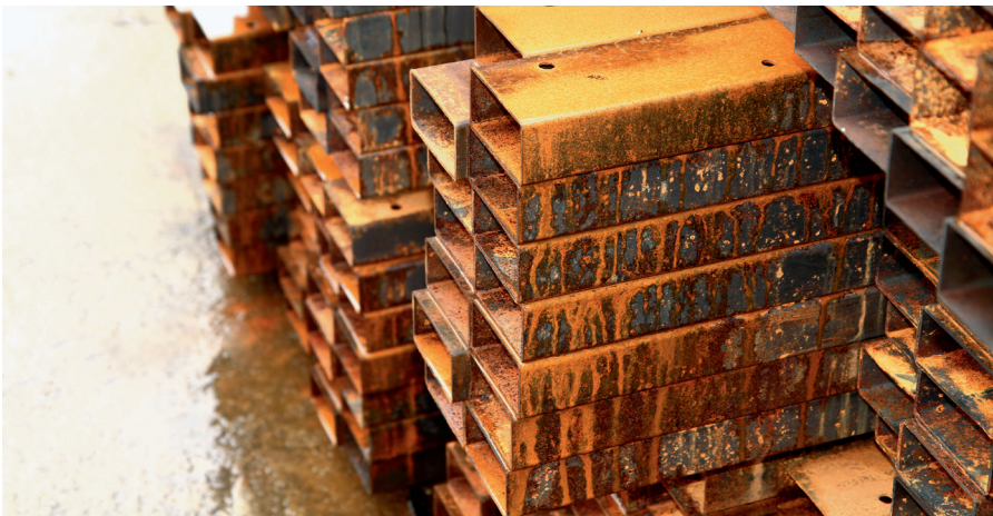
Fig. 4: Corrosion of steel components.
