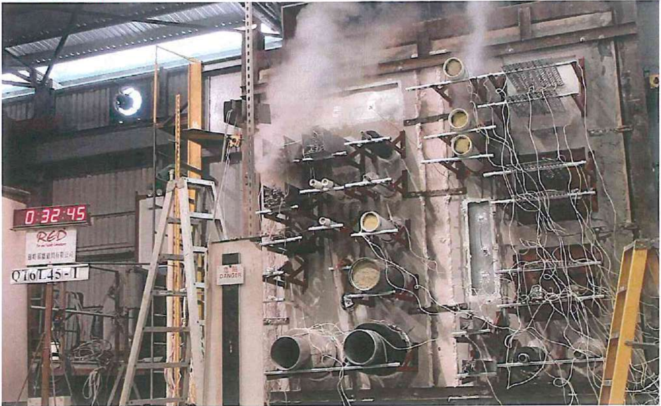
Photo 2: The unexposed face of the specimens after a heating period of 32 minutes.
